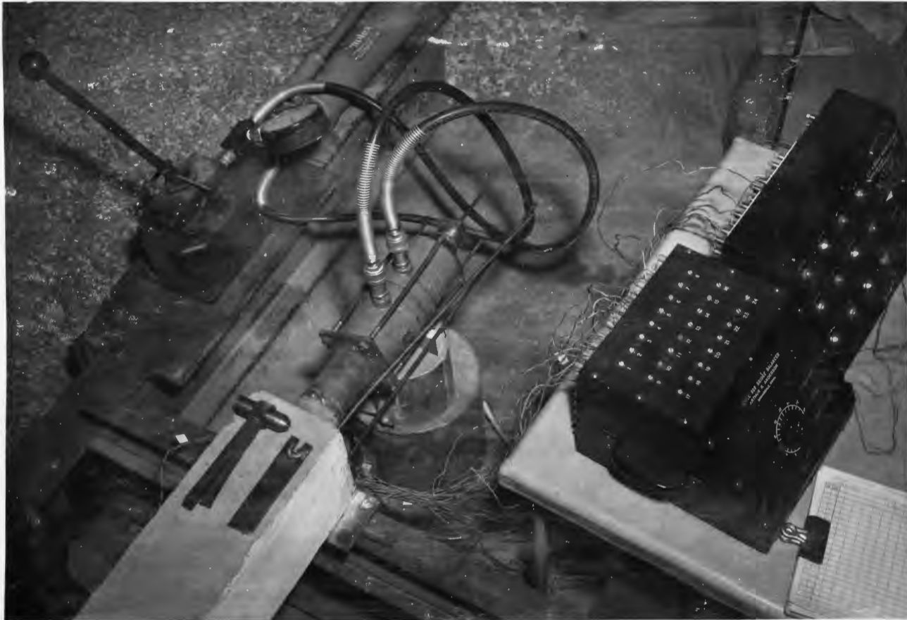
Fig. 26 Jacking unit in position for stressing a wire. Strain gage switching units at extreme right.
