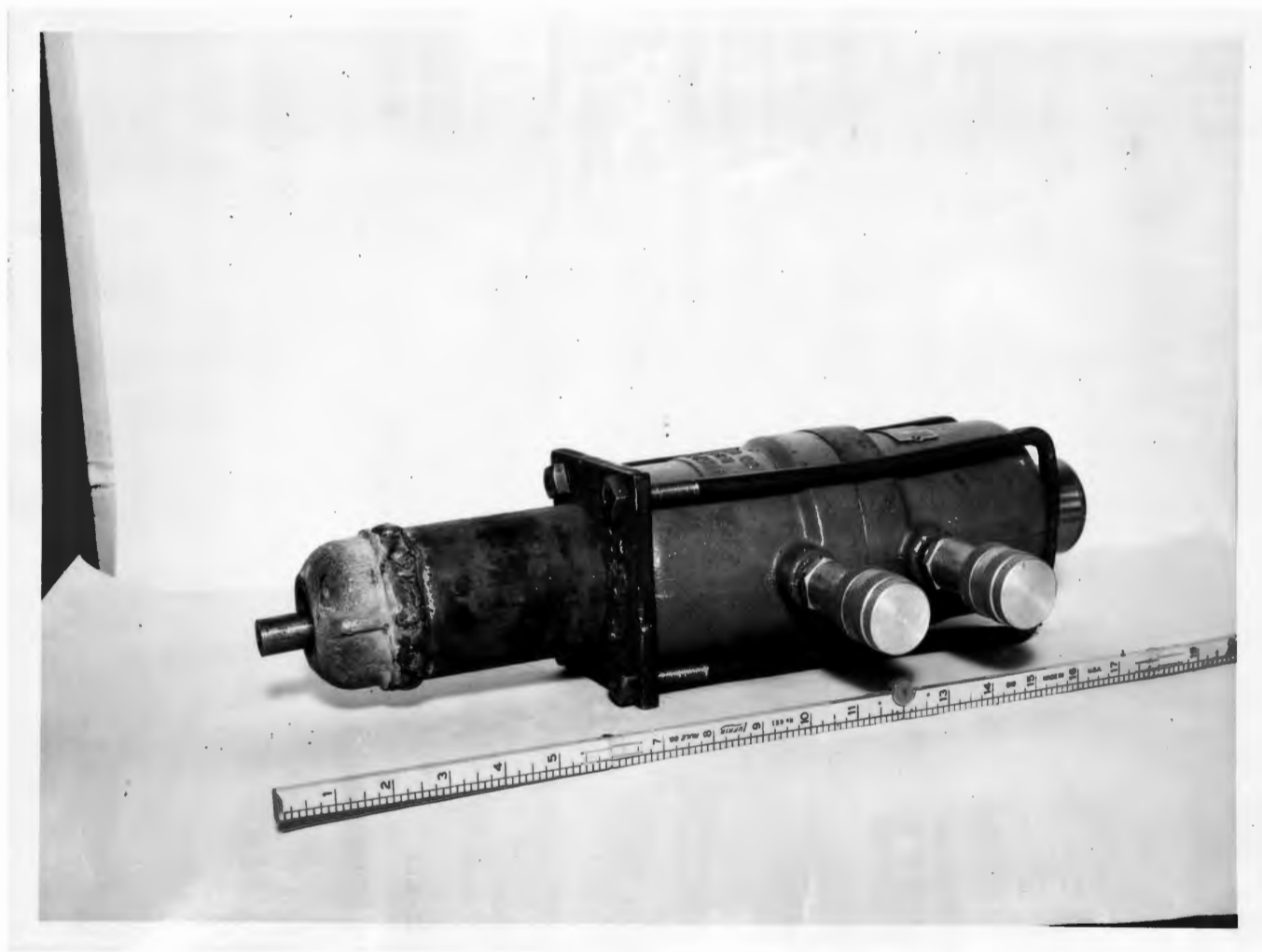
Fig. 24 Prestressing unit assembled.
