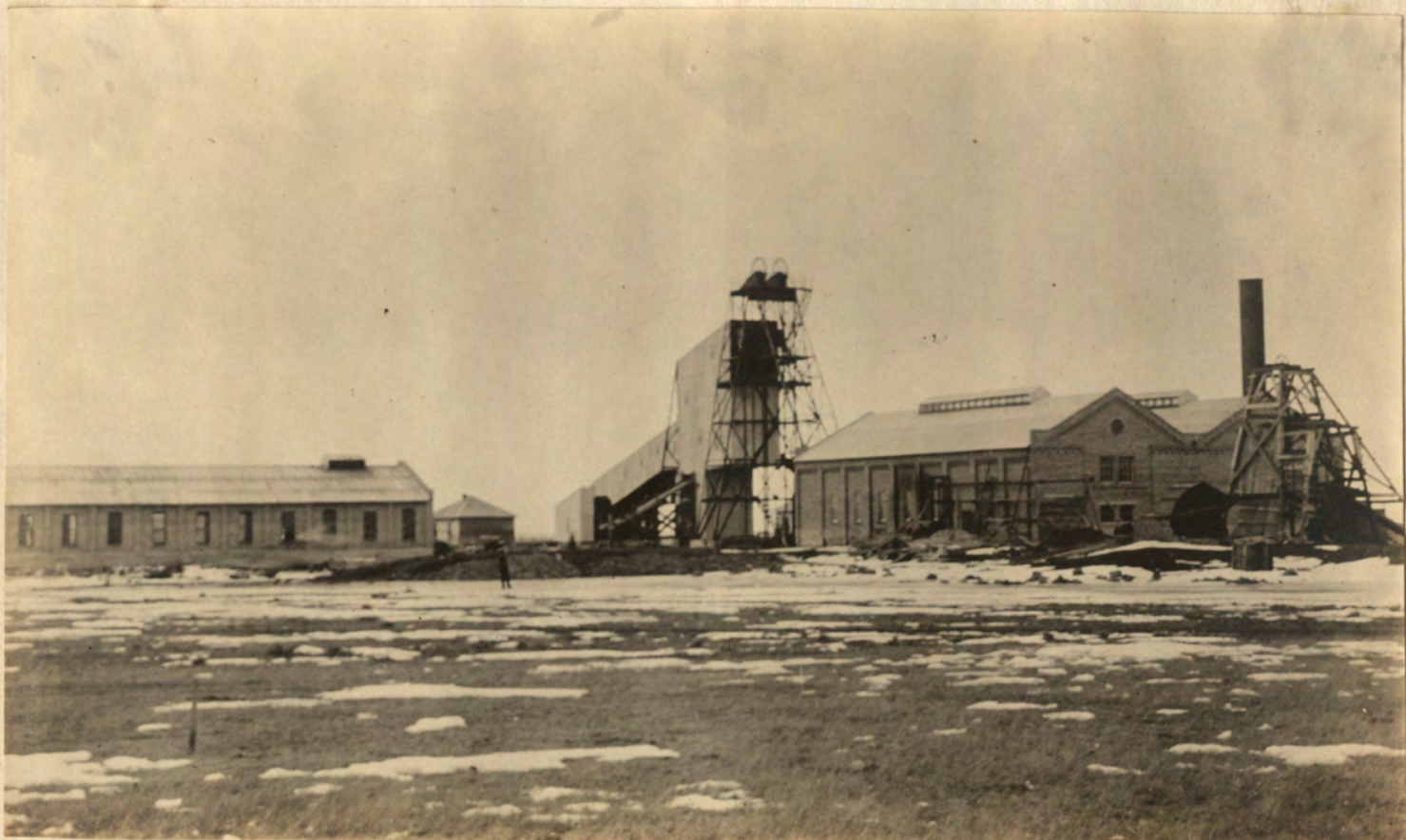
General View of Plant from the Southeast.
