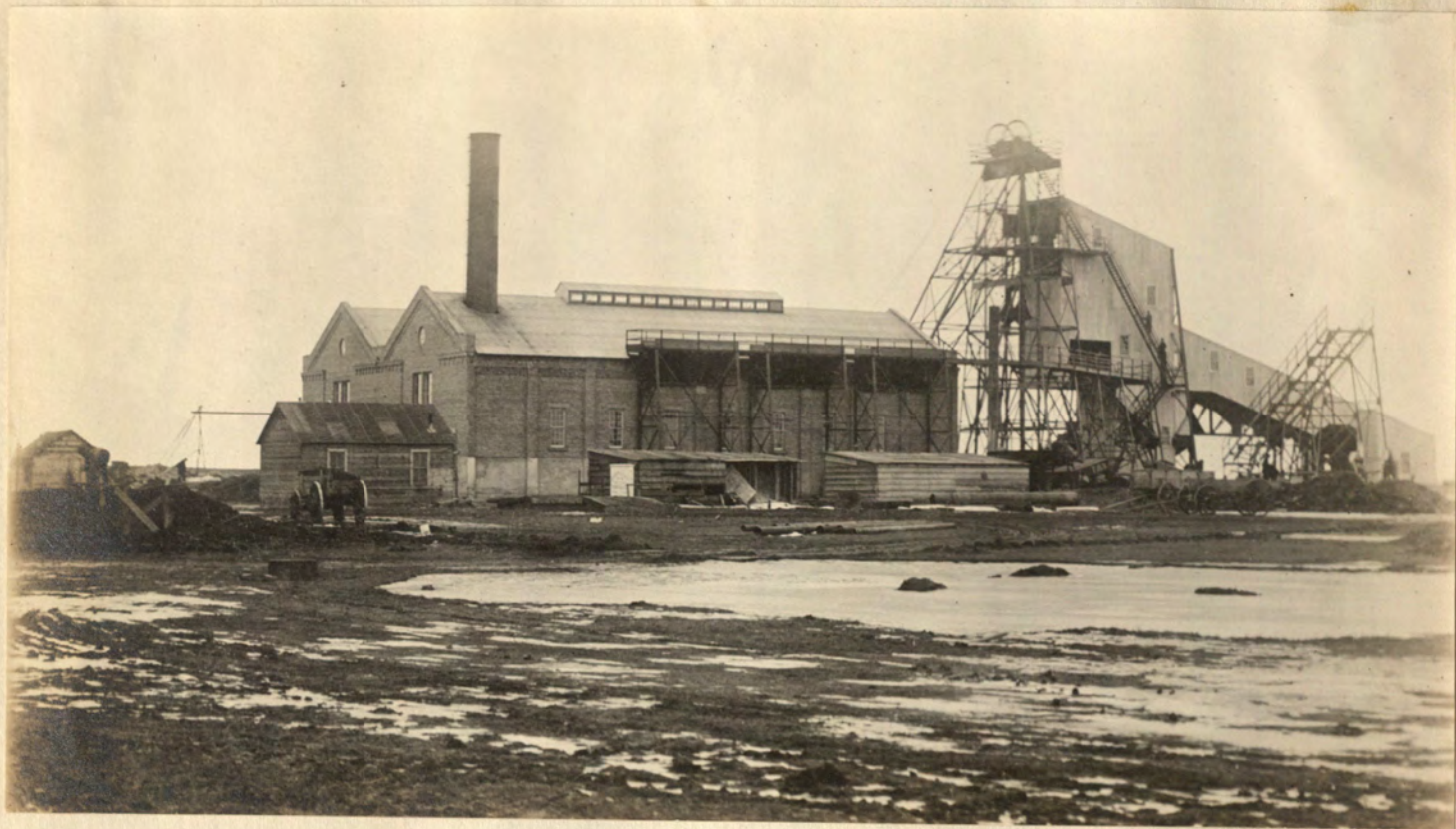
General View of Plant from the Southwest.
