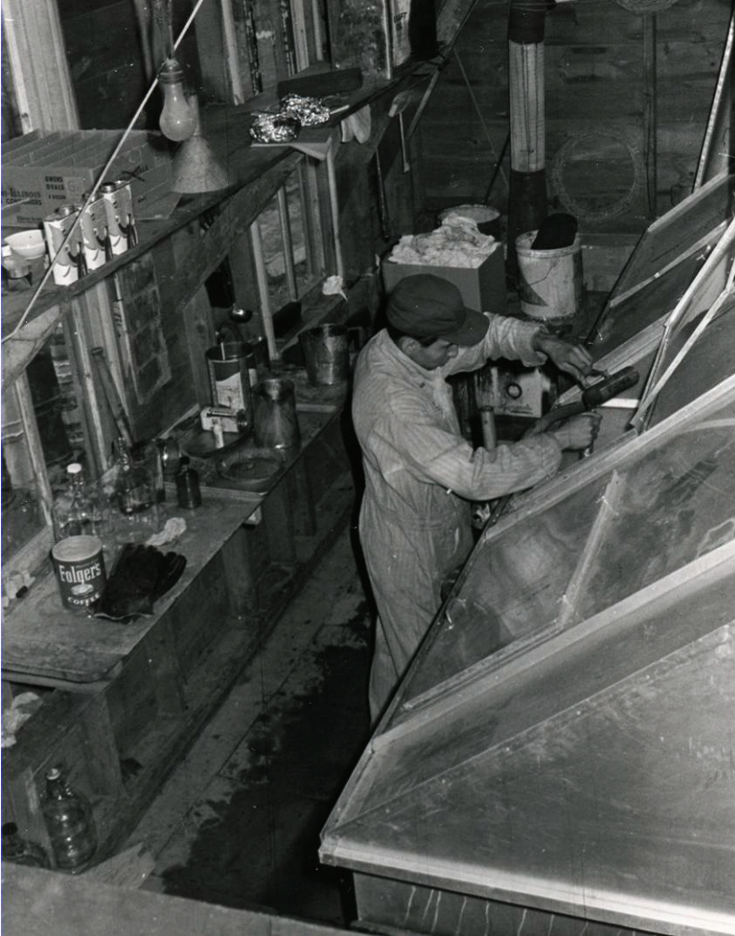
Figure 3. Brother John Anderl putting a log in the firebox of the evaporator in the original sugar house in 1955. Note that the stove is elevated about 16 inches. Image by permission of St. John's Abbey Archives.
