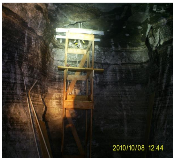
Figure 10. Wooden structure with aluminum plate to hold riser pipes.
