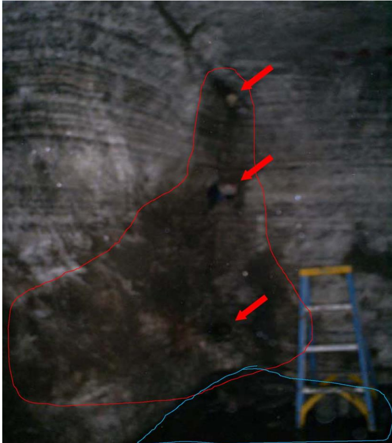
Figure 1. Red arrows indicate where the blast “boot holes” which intersected the abandoned well are located. The thin red line outlines the area along the “rib” affected by the water/mud spray following the blast that exposed the abandon well bore. The blue line outlines standing water left on the floor. The ladder is 1.5 meters’ high.
