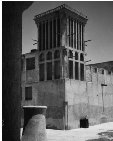
A wind tower in the Bastakia Quarter east of Dubai Creek in old Dubai. Open at the top on all four sides, wind towers caught the prevailing breezes and funneled the air down into the house for cooling the rooms below. Such wind towers were common along the coast of Iran. (Photo by Anna Lisa Ohm)
