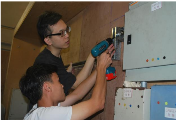
Electrical Installation Training in IVE (Haking Wong)
