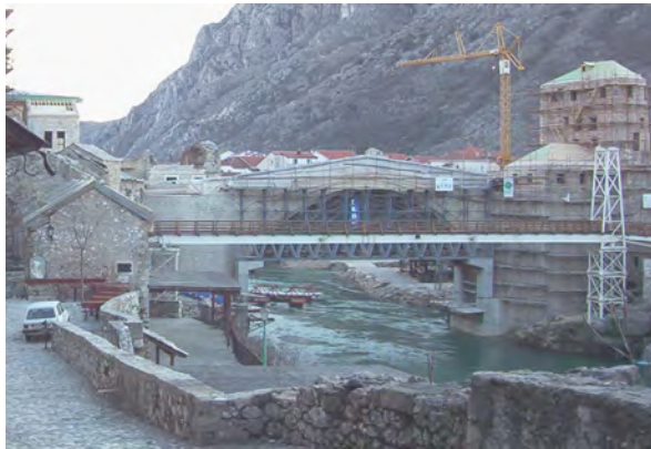
Figure 4.2. Photo image. Mostar bridge under construction in 2004. Copyright Alpha Woodward.
