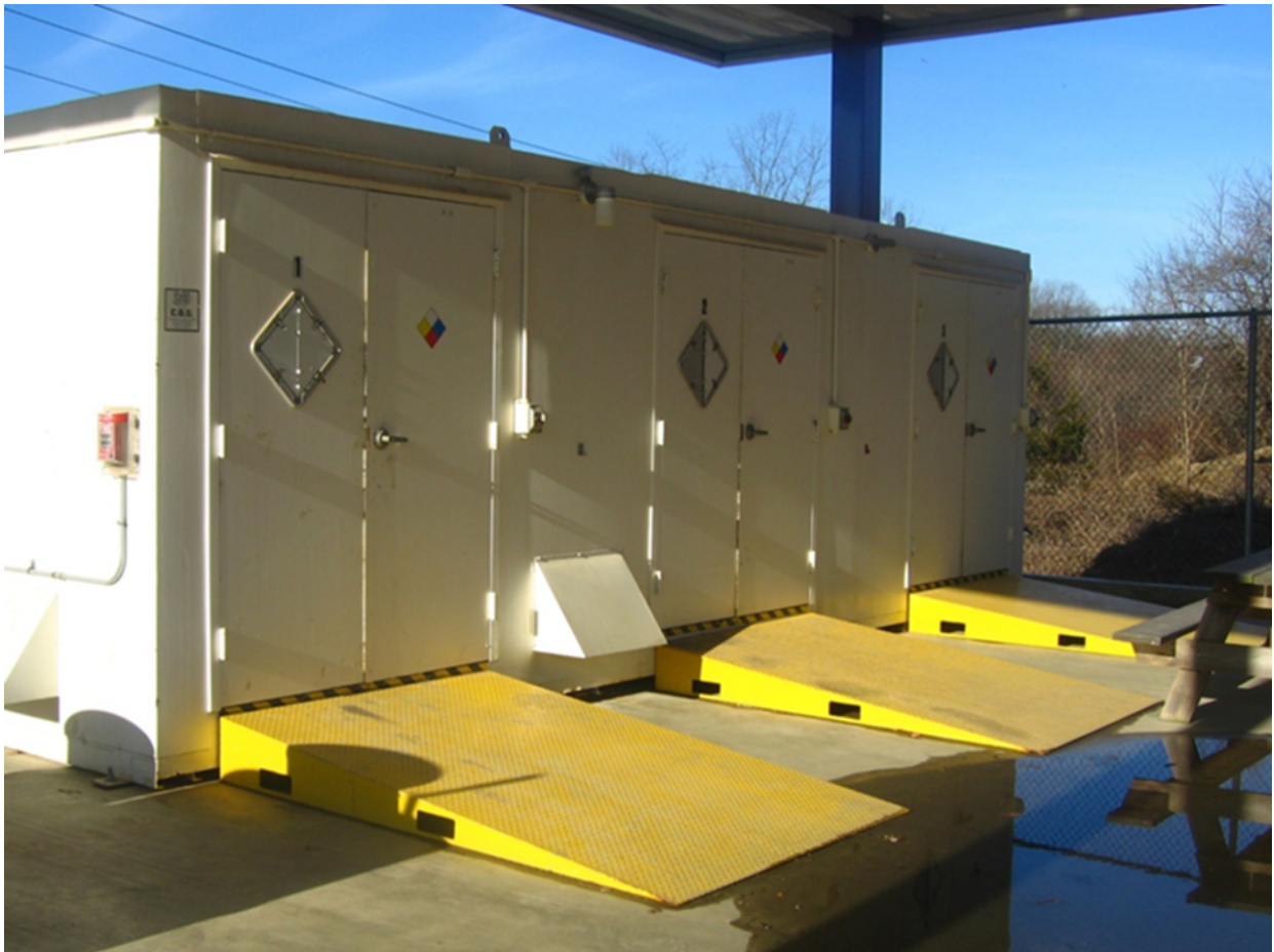
Figure 1. Permanent household hazardous waste facility storage building, Essex, CT. Photo by J. Ehle/Meyer. Reprinted with permission from Connecticut River Valley Council of Governments (River COG), Essex, CT.
