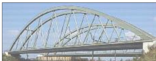
FIG. 2 Landegem railway bridge.
