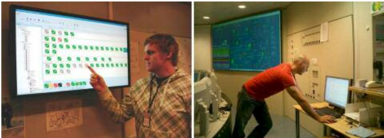
FIG. 6 Sand Management software installed in the product optimization room and platform control room at the operator. The screen shows the status of each sand probe by colour code.
