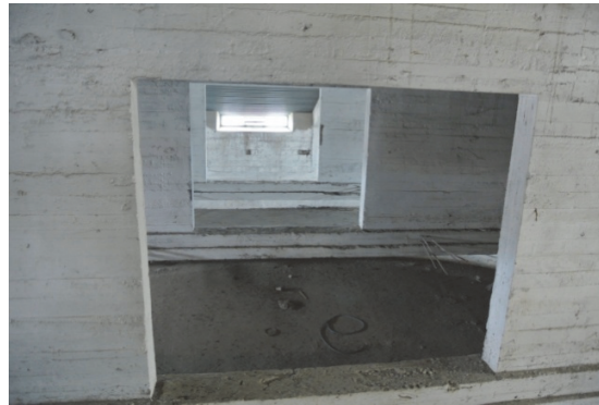
Figure 12: The extrados of the vault of the "Sala Camuccini".
