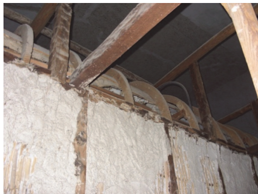
Figure 11: No-load-bearing masonry vault composed of timber skeleton visible from the Library.
