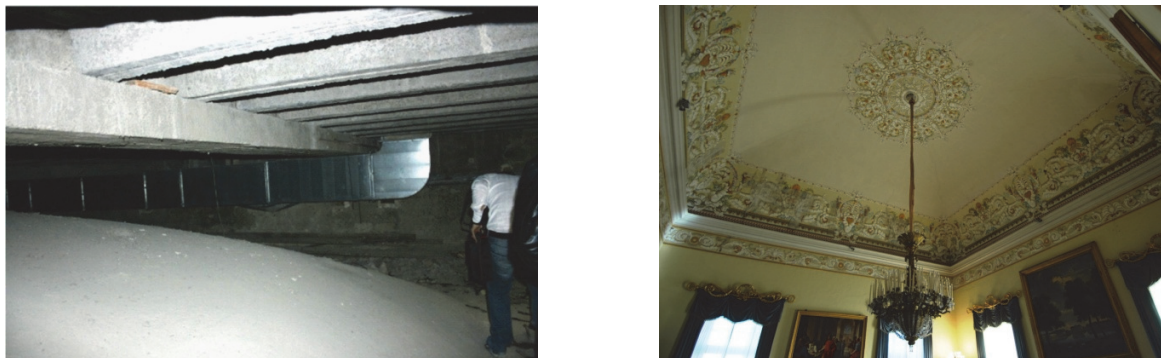
Figure 10: No-load-bearing masonry vaults with overlying horizontal diaphragm: the "Sala della culla".
