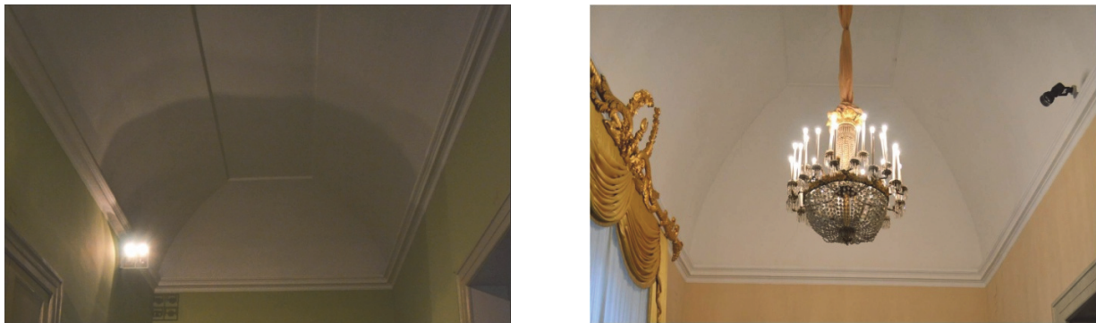
Figure 9: Load-bearing masonry vaults.
