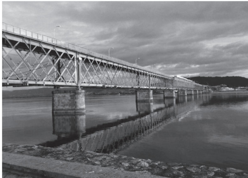
Figure 5: Riveted metallic Eiffel bridge in Viana do Castelo (Portugal).
