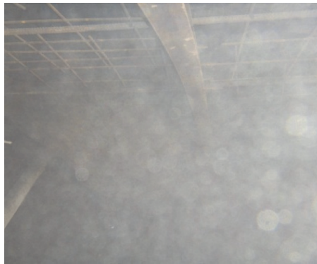
Figure 13: Field dry-mix shotcrete.
