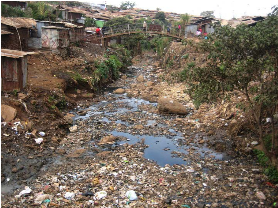
FIGURE 12: Refuse in Drainage Channel in Slum Area
