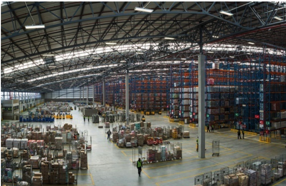
Shoprite Distribution Centre in Cape Town
