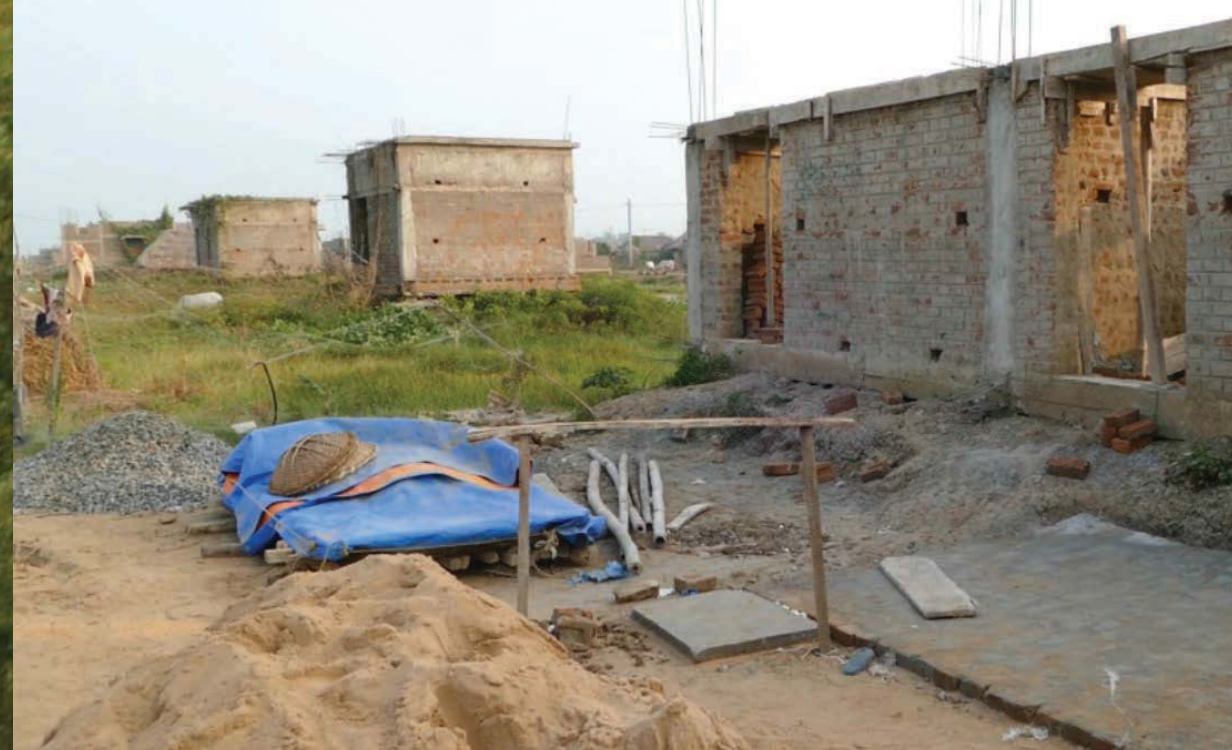
Houses under construction in Bagapatia.
