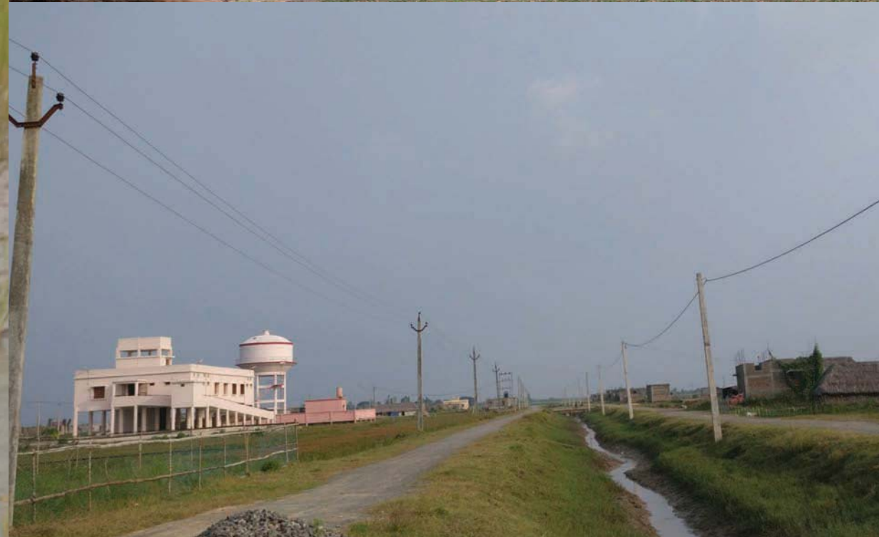
Overhead tank for drinking water, cyclone shelter, and electrical lines at Bagapatia
