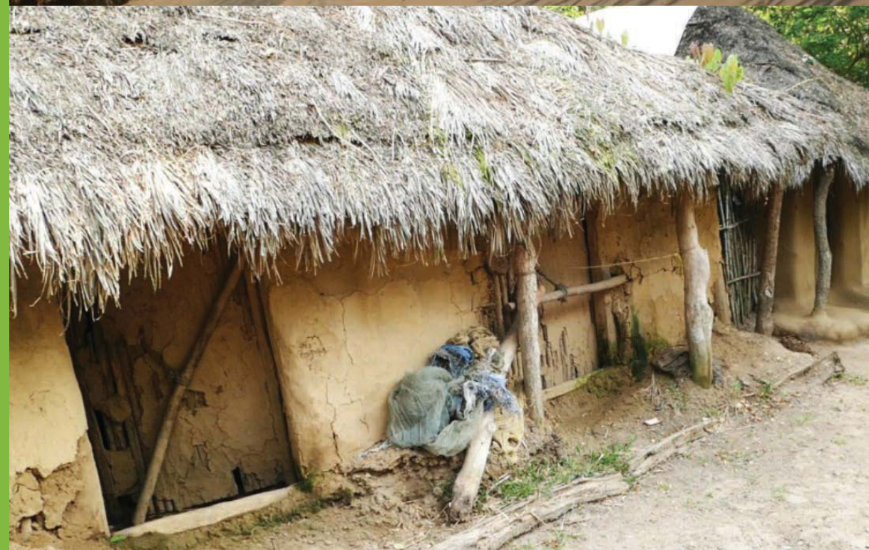
Traditional “kutcha” houses made of mud and thatch are easily eroded and damaged by floods
