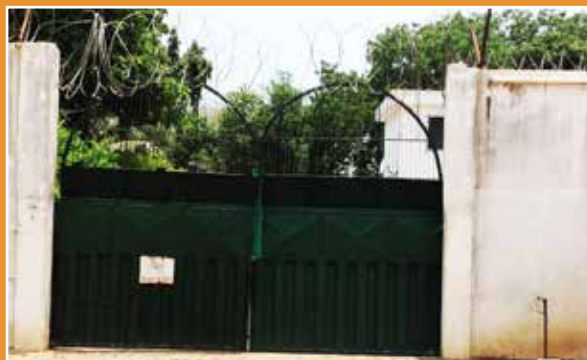
High fence wall with barbed wire
