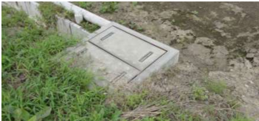
Photo. 5-1 Sedimentation tank around A swamp
