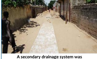
A secondary drainage system was constructed in the neighbourhood of Al Pulaar in Yeumbeul North, which has helped to reduce flooding
