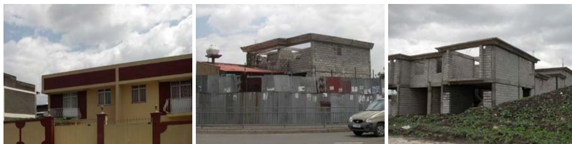
fig 56 – Private built concrete houses in Addis Ababa. (Pictures Tjerk Reijenga)
