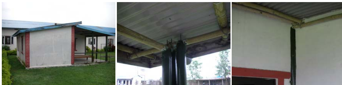
fig 35 – Bamboo house in Hetauda at the Himalaya Bamboo Pvt. Ltd.. (Pictures Tjerk Reijenga)
