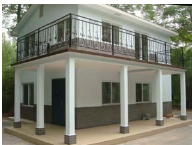
fig 3 – The Black Bamboo Garden house fully constructed with bamboo panels but with a nice and temporarily look. (Pictures Tjerk Reijenga)
