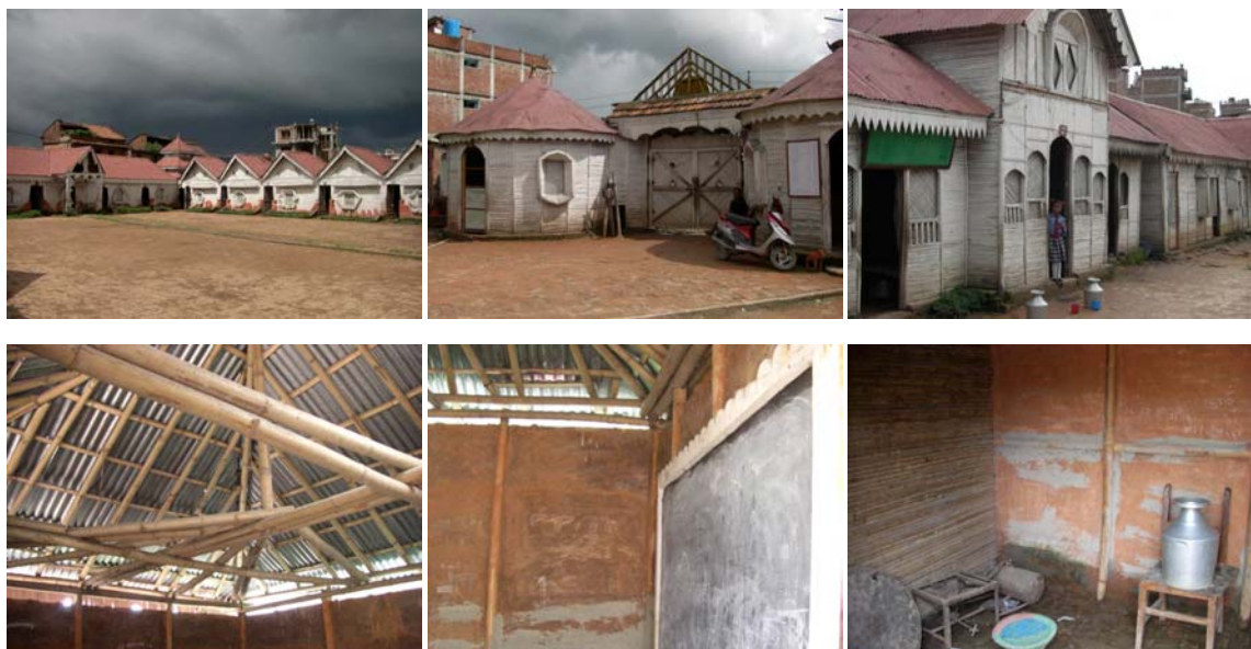
fig 34 – Bamboo school building in Thimi close to Bakhtapur. This construction is plastered with mud on the inside. (Pictures Tjerk Reijenga)
