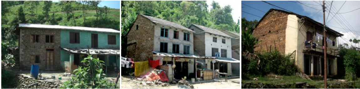
fig 31 – Recent masonry houses along the road between Kathmandu and Pokhara (Pictures Tjerk Reijenga)
