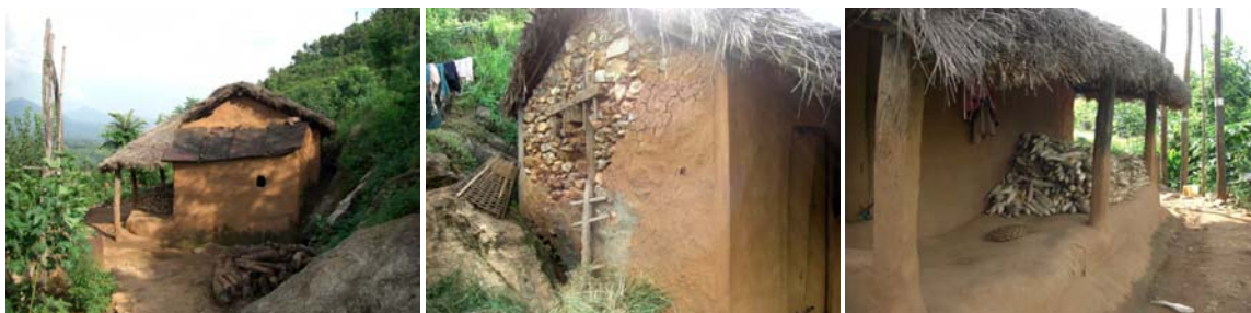
fig 30 – Traditional masonry houses near Bandipur (Pictures Tjerk Reijenga)
