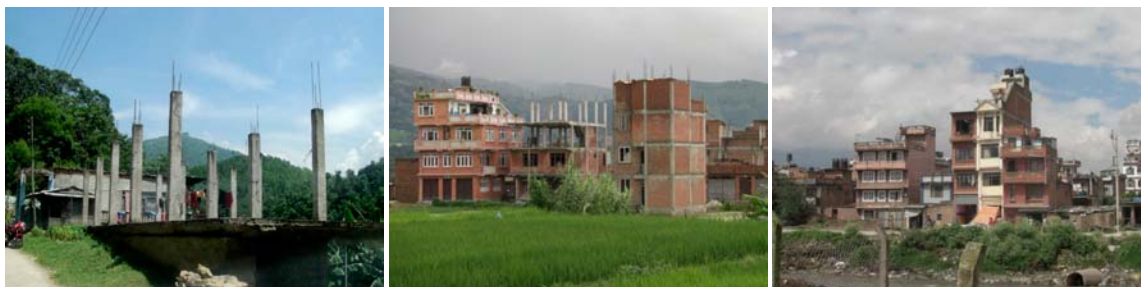
fig 38 – Private built concrete and masonry houses in Kathmandu Valley. The construction is a long process by adding terraces and volumes. (Pictures Tjerk Reijenga)
