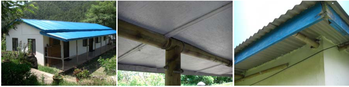
fig 36 – Bamboo house in Baireni. One of the first of this type. (Pictures Tjerk Reijenga)
