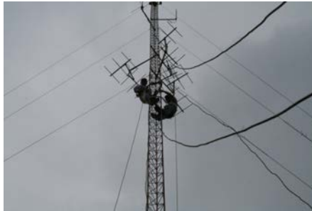
Figure 2. Installation of the telecommunication node
