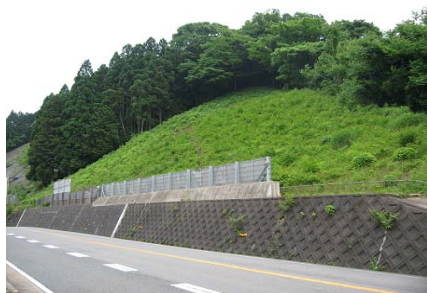
Figure-3. View of the non-support slope (area-B)
