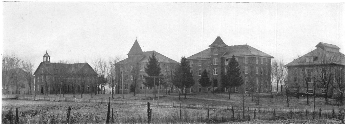
MAIN GROUP OF BUILDINGS
