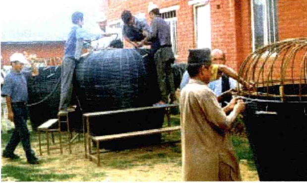
Plate 4.6.1 Construction of roofwater harvesting jars for drinking water.
