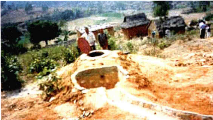
Plate 4.6.3 Underground cistern to collect monsoon runoff to be used for irrigation
