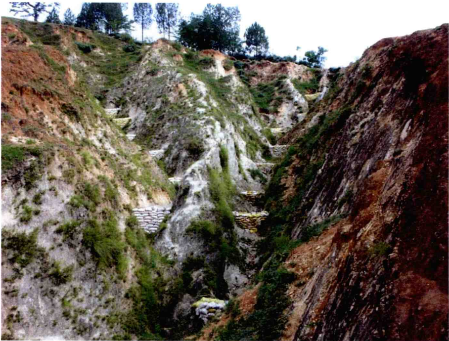
Plate 5.2.2 Gully stabilization at Dhotra site
