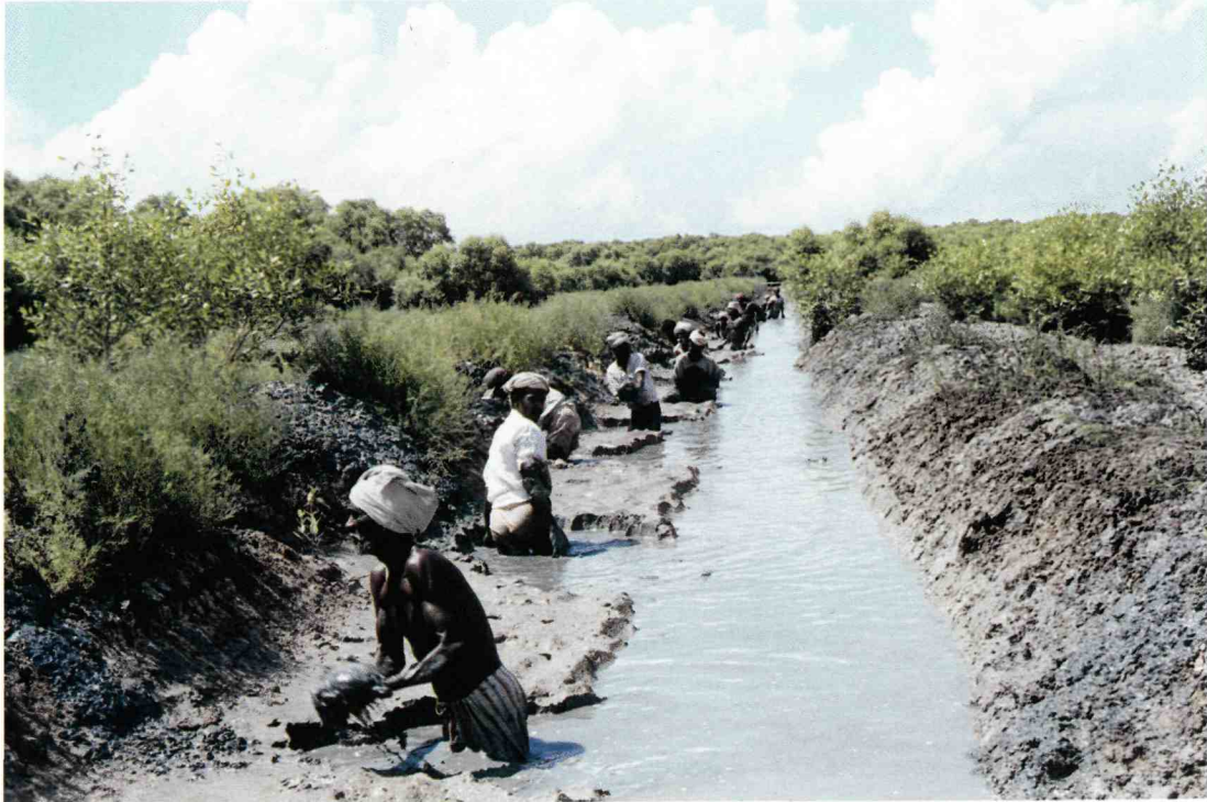
Figure 3.15 a. Desilting of the canals is one of the important tasks of mangrove management
