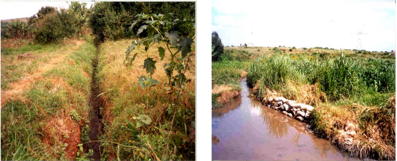
Figure 11: Hand dug canal and water diversion system using sand bags
