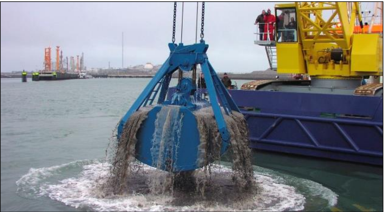
Figure 5-3. Mechanical dredging equipment (Royal IHC)
