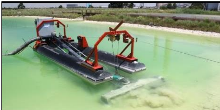
Figure 5-2. S.A.M.E. auger dredging, Australia
