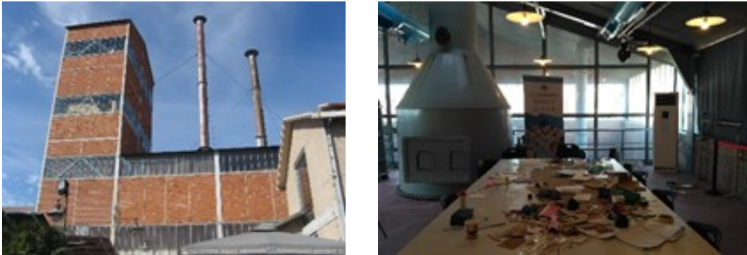
Figure 1. The informal pilot site in the Technopolis City of Athens.
