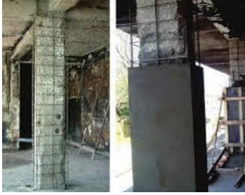
Fig.1.1. Concrete Jacketing of Column.
