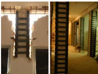
Fig.2.1. Steel jacketing of column
