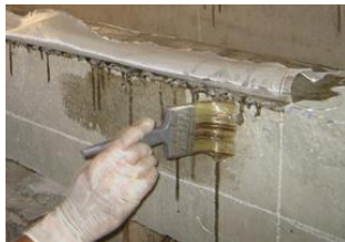
Fig.4.2. Application of epoxy and hardener on the beam.
