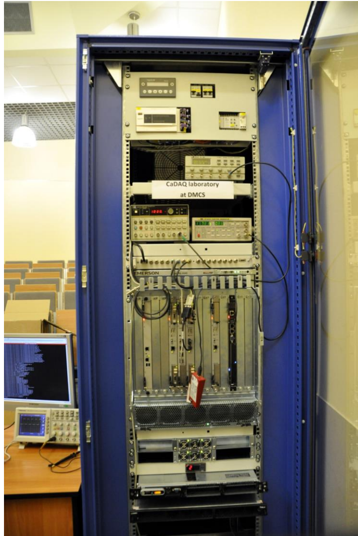
Fig. 18 Hardware installed in the ITER cubicle – front view
