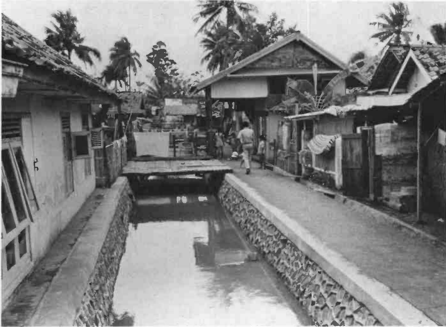
Improved drainage canal in Kampung Improvement Program site, Jakarta, Indonesia.
