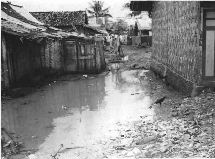
Drainage canal prior to the implementation of the Kampung Improvement Program, Jakarta, Indonesia.
