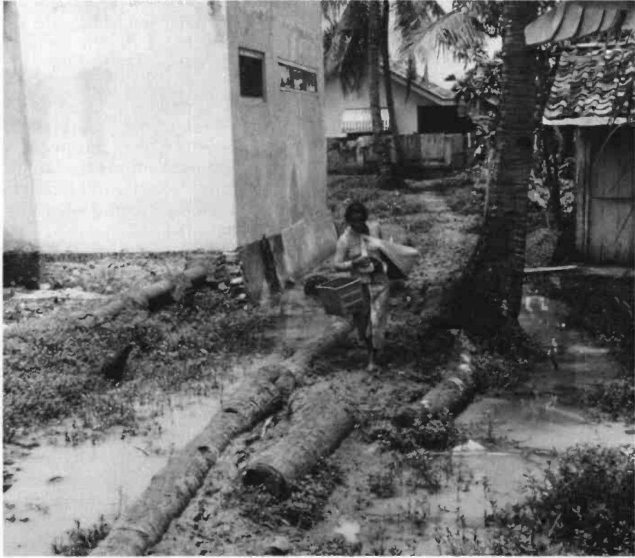
Walkway prior to the implementation of the Kampung Improvement Program, Jakarta, Indonesia.
