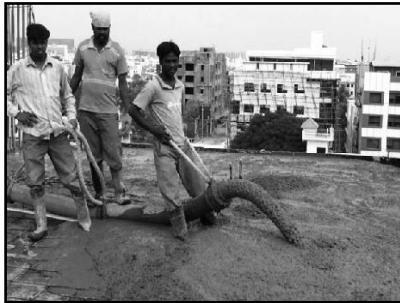
Fig.2. Concrete pouring
