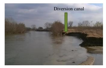
Fig. 4 River bed erosion and collapsed water intake
