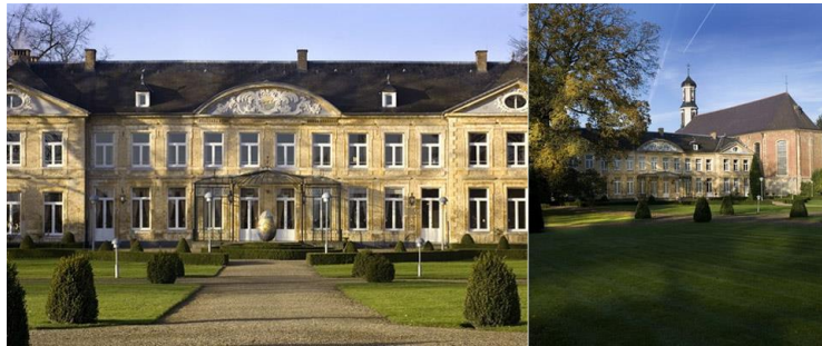
Fig. 1 Saint-Gerlach Hotel, Maastricht, Netherlands
