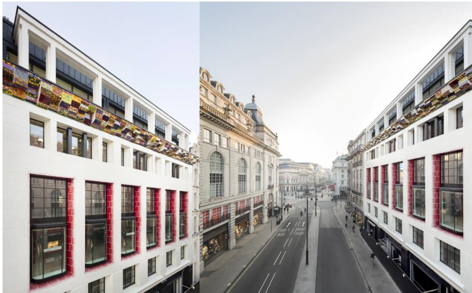
Fig. 3 The white faience facade fronting One Eagle Place, in London's Piccadilly, is adorned with a jazzy ceramic cornice by artist Richard Deacon and red window reveals; photos Dirk Lindner [12].
