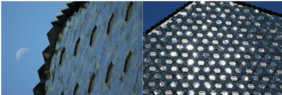
Fig. 2 Herzog & de Meuron has added a new roof to Basel's Museum der Kulturen, whose 3D tiles animate it, especially in strong sunlight. The steeply angled roof deliberately echoes the rooflines of the surrounding medieval buildings [12].
