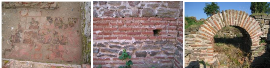
Fig. 5 Usage of bricks for floor tiles and wall construction at an early Byzantine site, Iustiniana Prima (6 th century) in Serbia. Photo A.Momčilović Petronijević and Ć. Vasić
