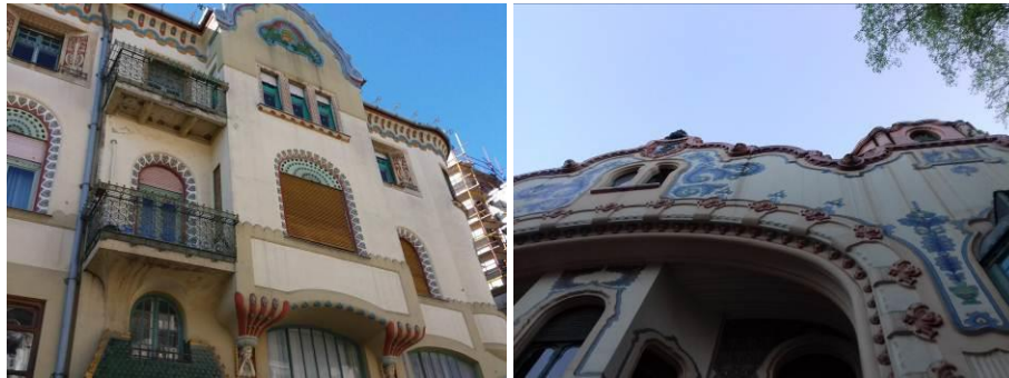
Fig. 10 Usage of ceramic elements in façade decoration, Subotica, foto A.M.Petronijević
