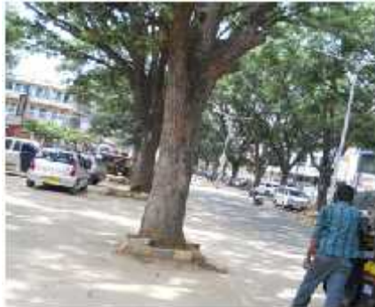
Plate 20. Lack of aeration and watering to the roots – 1 st main in Saraswathipuram.
