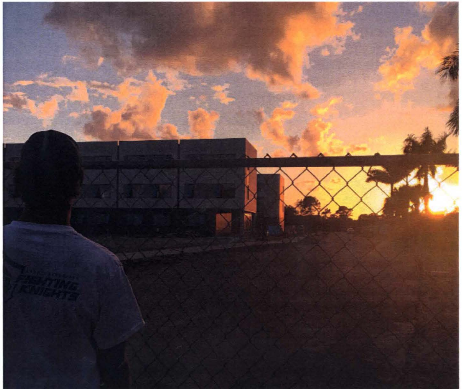
Above: Thomas Wagner, junior, overlooks the progress being made to the new residential building. Staff Photo / C. Kruse.
