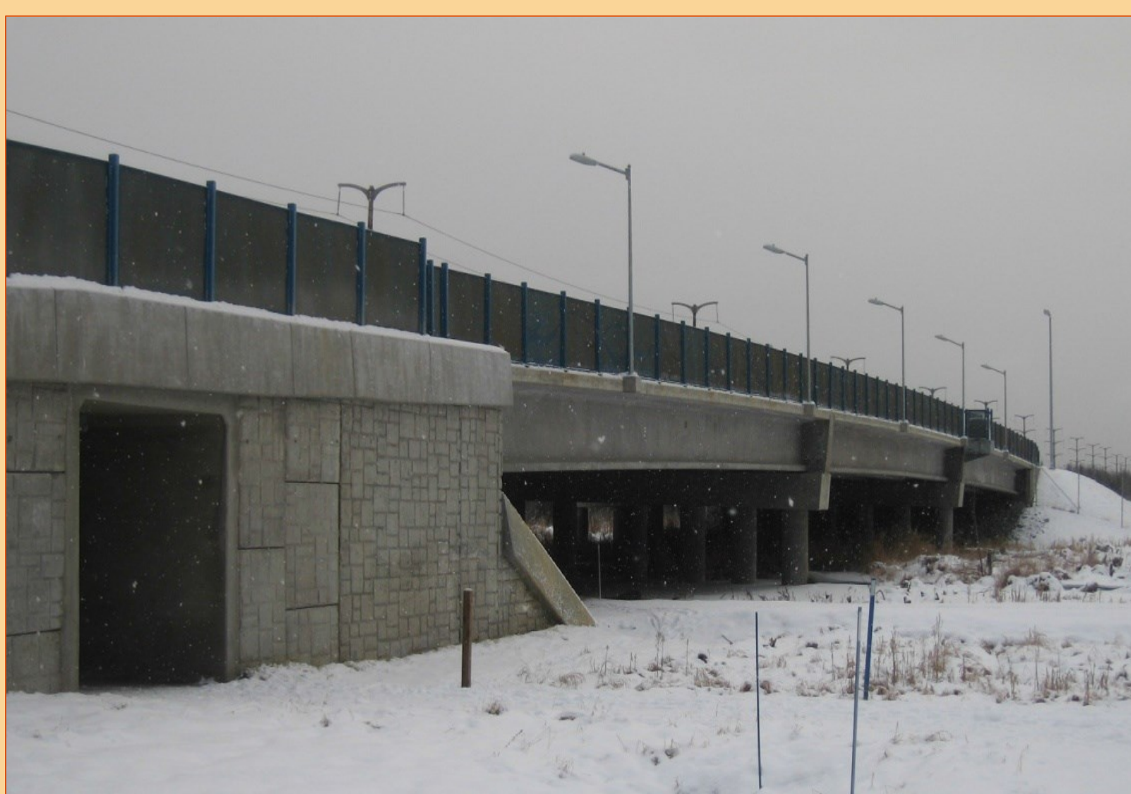
Figure 1: Campbell Creek bridge main view
