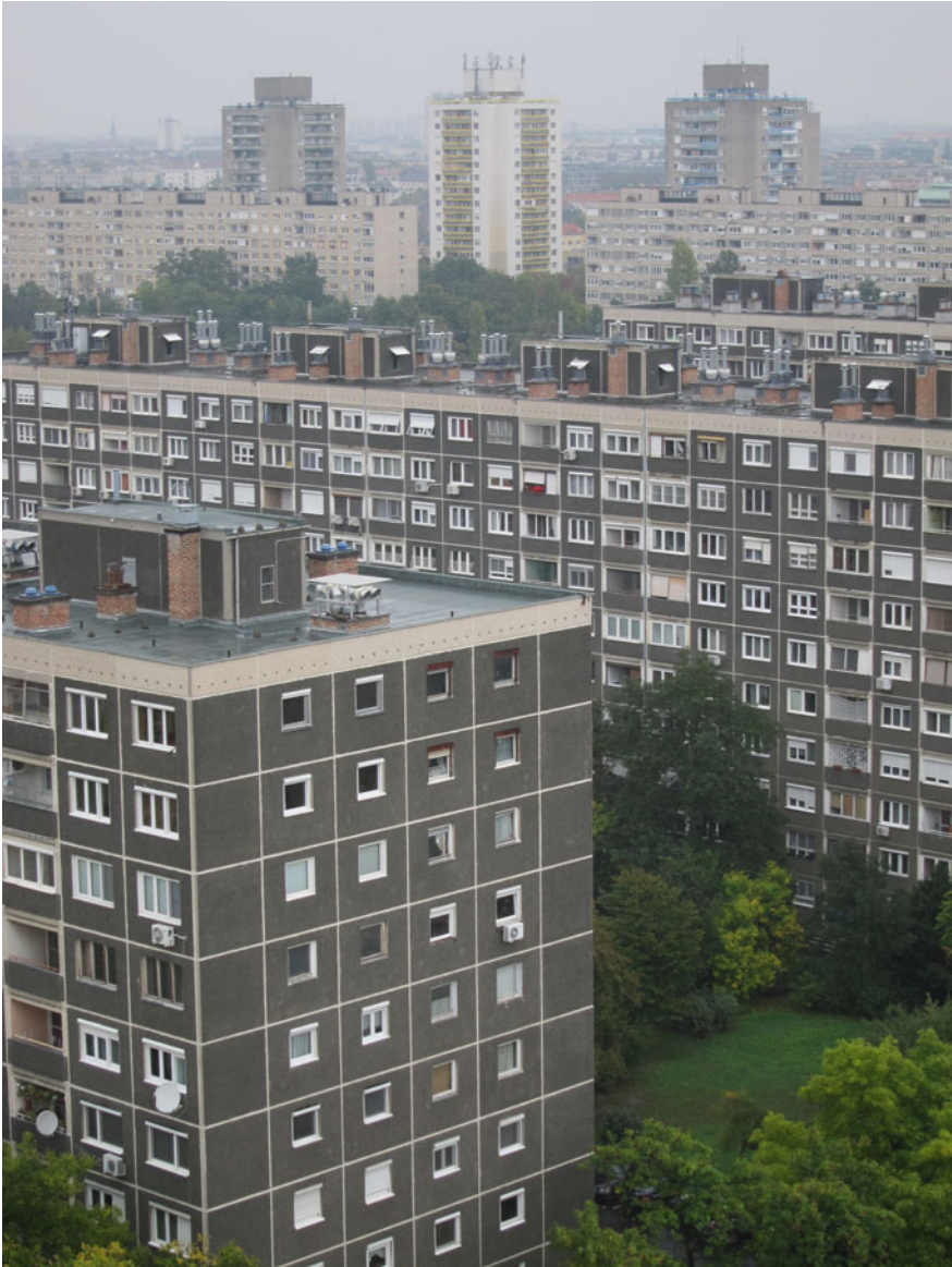
Fig. 6.2 Kelenföld, Budapest: pioneering prefabricated blocks built from 1965 using a Soviet spin-off of the Camus system Source M Glendinning, 2015
