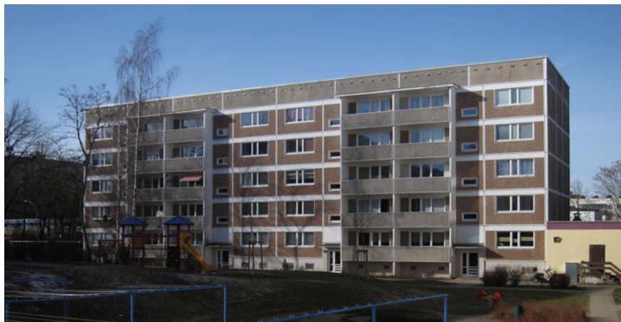
Fig. 6.3 Koszalin Str. 1-7, Neubrandenburg, East Germany: the first built example of the GDR's WBS 70 standard large-panel prefabricated concrete series, constructed in 1973 (and designated a heritage monument in 1984) Source M Glendinning, 2017
