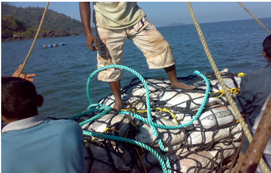
Figure 4: Single point mooring using sand filled bags (Gabbion box)
