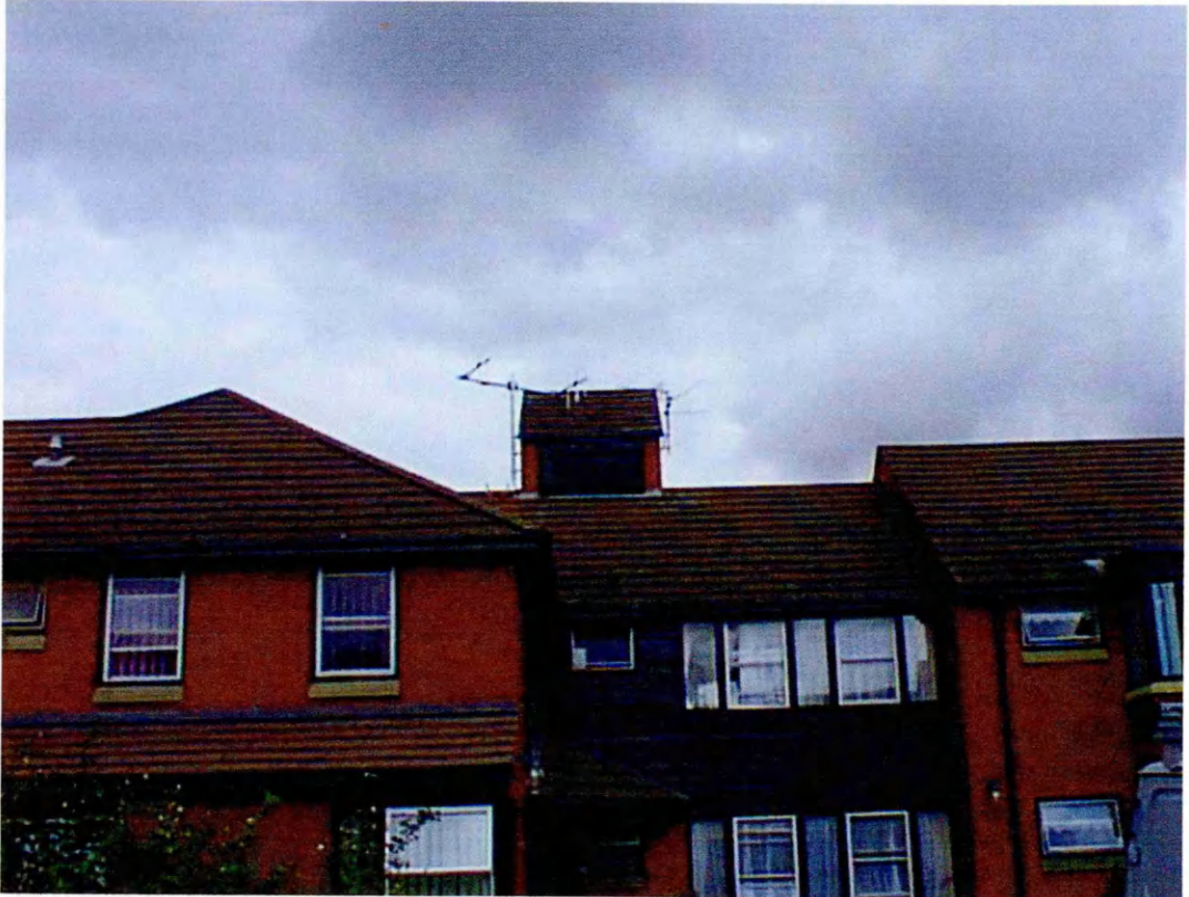
Figure 53 Prospect House Day care centre with Dual Yagi antennas
