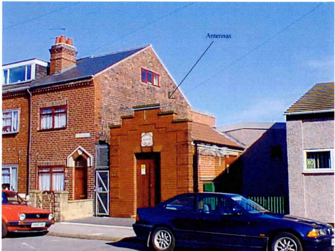
Figure 56 Queensway Electricity Sub Station
