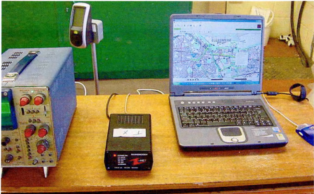
Figure 37 Nimbus Mk1 PLM Transmitting in Training Ground Sub-Station
