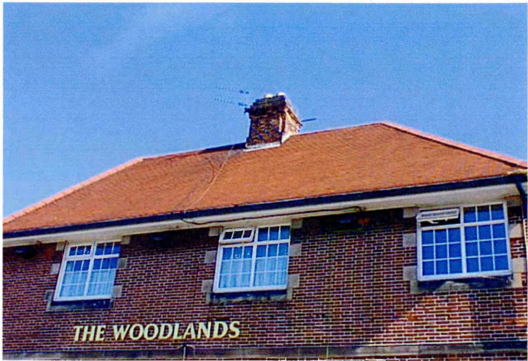
Figure 55 Woodlands Public House Node showing twin Yagi antennas
