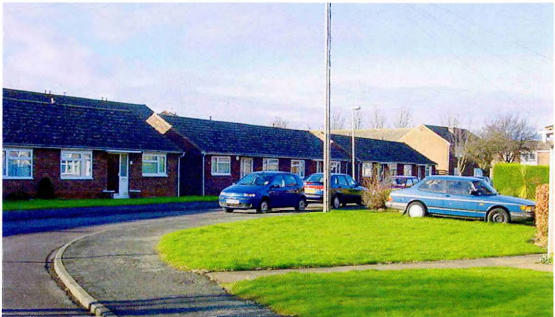
Figure 73 Belverdere Crescent again showing the spaces between buildings and low roofs
