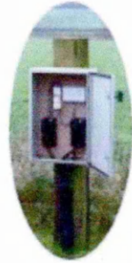
NIMBUS PLUG-IN AND OSCILLOSCOPE MONITOR POINT
