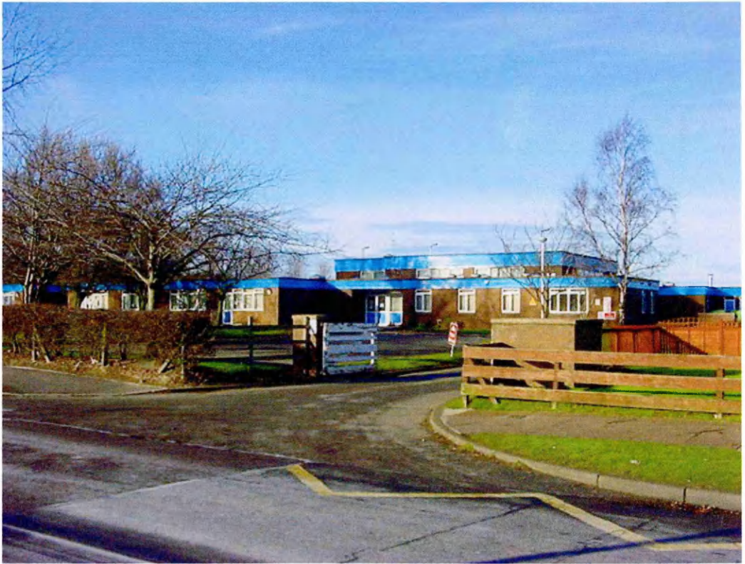
Figure 70 Parkside Primary School
