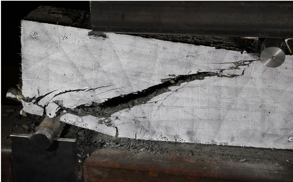
Figure 6-8 Failure in shear
