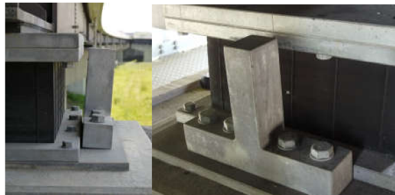
Figure 2-16: Deformation of the bearing stopper of the consecutive span
