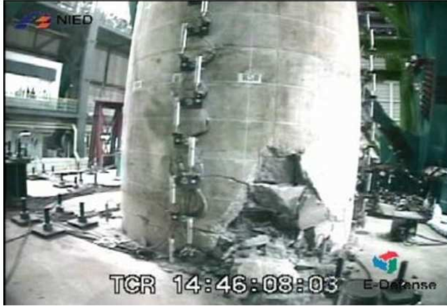
Figure 6-66: Damage to RC pier after 1st 100% Takatori excitation [1] (2007-1213-004-1M)
