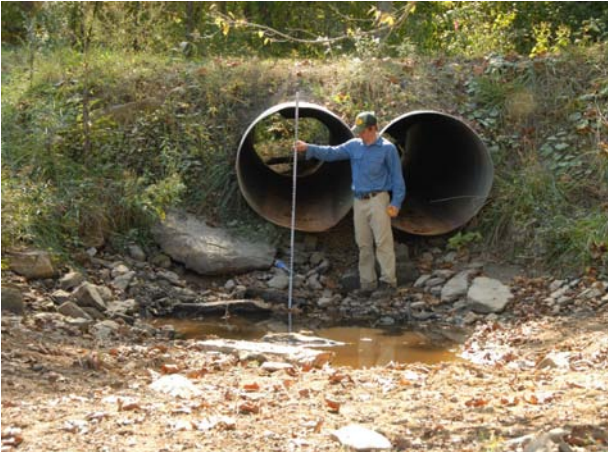
Figure 5. One of two pools in the pre-restoration Mill Branch channel that provided refuge for the threatened blackside dace during the summer and fall drought of 2008.
