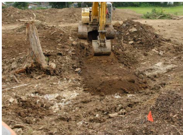
Figure 8. Small groundwater dam constructed at riffle.
