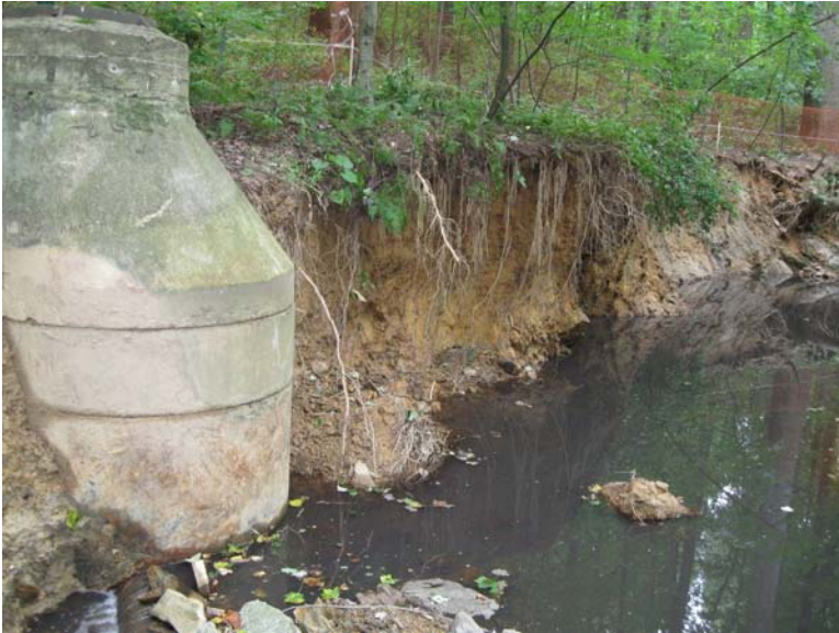
Exposed sanitary manhole.
