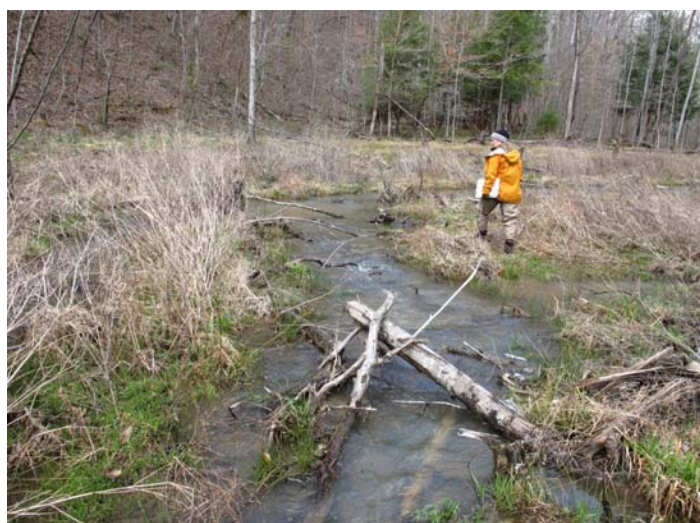
Figure 4. Slabcamp Creek restored valley bottom and channel reestablished on pre-settlement gravels. Photo taken approximately one year after construction.
