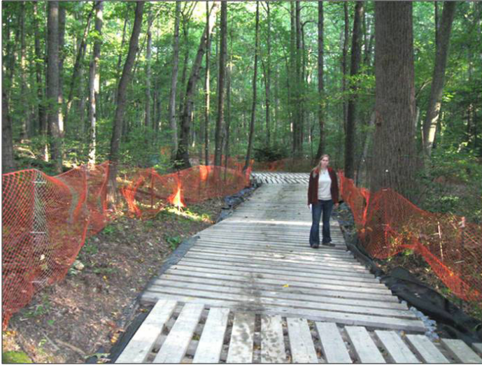
Timber deck mats along access path in The Glade .
