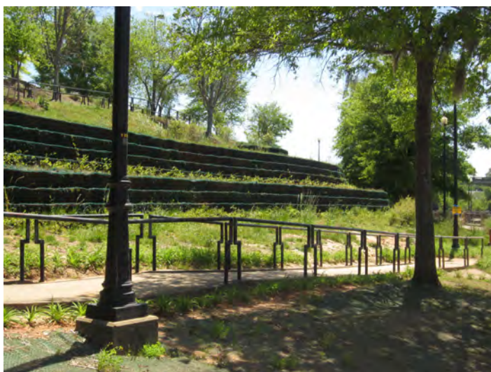
Figure 5.: Two examples of stabilization along Riverwalk.
