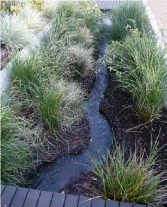
Vegetated swales planted along roadways can absorb stormwater to help prevent sewer overflows. Source: EPA, Nancy Arazan ( https://www.epa.gov/sites/production/files/2015-11/documents/sw_ms4_compendium.pdf )
