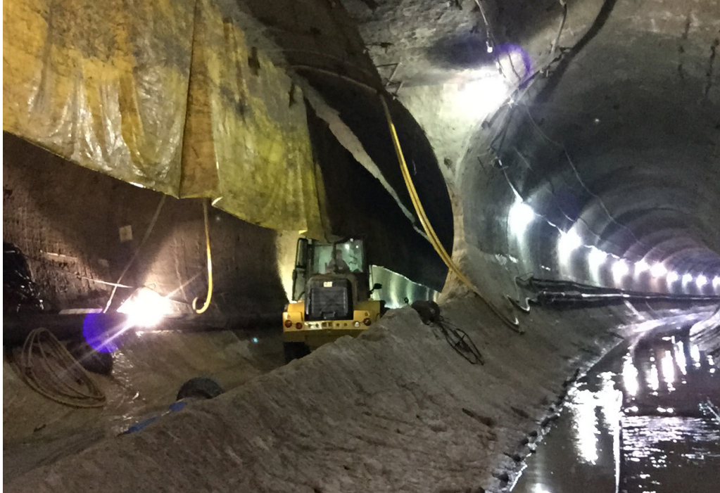
Deep Rock Tunnel Connector
