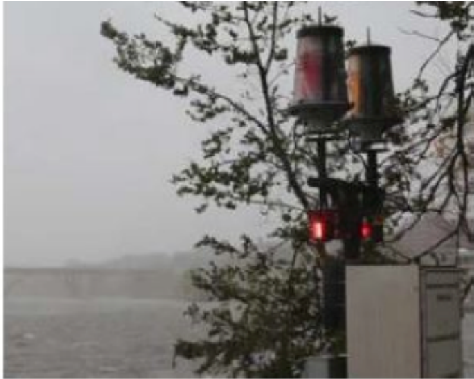
Washington, D.C., was required to place a CSO indicator light at several CSO outfalls along the Potomac River as part of their CD. Source: EPA ( https://www.epa.gov/sites/production/files/2015-06/documents/npdesnextgencomplcompendium.pdf )
