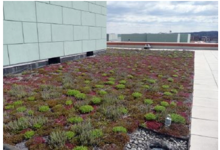
Planting gardens on rooftops is another type of green infrastructure that can reduce the impact of wet weather events on sewer overflows. Source: EPA, Nancy Arazan ( https://www.epa.gov/sites/production/files/2015-11/documents/sw_ms4_compendium.pdf )
