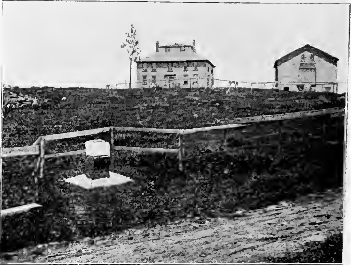
Old Fort House, Barn, and Tablet Inscribed: "A Large Number of Cannon Balls Fell in This Vicinity."
